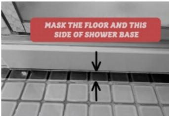
Then, stick masking tape down Line A so it goes up the tub about 1/8 in.
